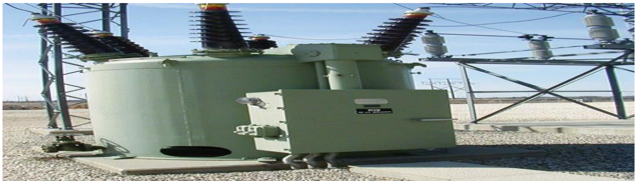
Outdoor medium voltage oil-immersed circuit breaker
